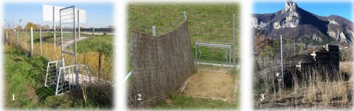
Examples of escapes route: 1) boar hatch Sanglipass, 2) tilting trapdoor, 3) deer ramp Photo credits: 1) and 3) Cabinet X-AEQUO, 2) JF BRETAUD - CEREMA Ouest
