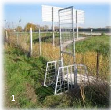
Examples of escapes route: 1) boar hatch Sanglipass, 2) tilting trapdoor, 3) deer ramp Photo credits: 1) and 3) Cabinet X-AEQUO, 2) JF BRETAUD - CEREMA Ouest
